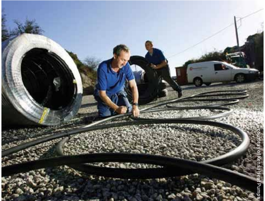
Groundsource heat pump installation
